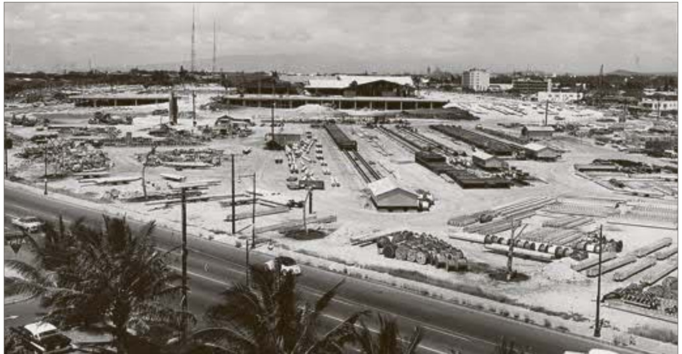
ABOVE: A temporary concrete plant was built in 1957 on the diamondhead end of the construction site, next to Atkinson Drive, to speed the construction time of building Ala Moana Center. This site was later the second phase expansion of the center with Liberty House and J.C. Penney, which opened in 1966.
